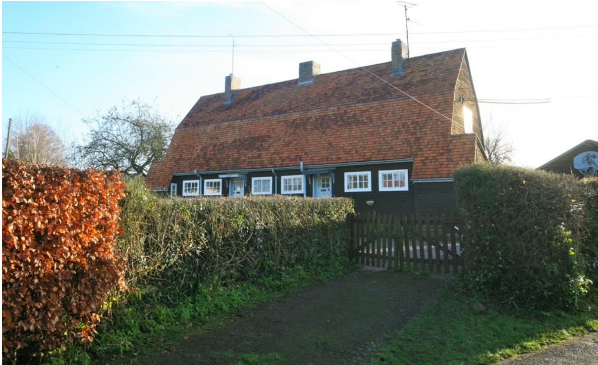
Fig.51 Plas-yr-Haul, an unusual timber-clad estate property with cedar shingle roof
