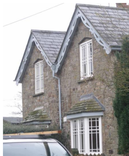
Fig.61 An attractive, well preserved pair of semi-detached cottages of the first half of the 19 th century which incorporate many of the rustic/romantic features of the cottage ornée style, whilst being quite formal in plan.
