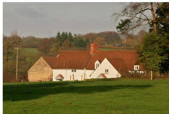
Fig.16 White-washed stone buildings are a feature of Argoed Farm
