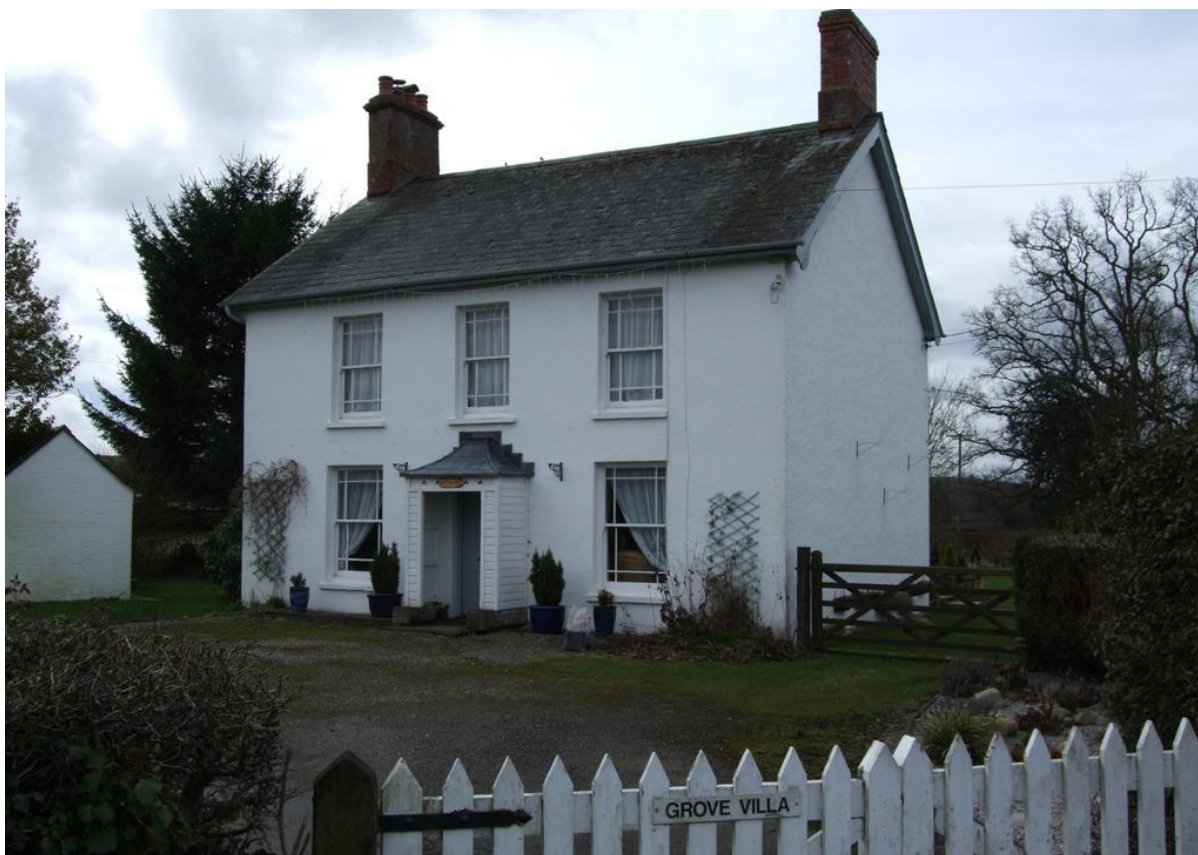
Fig.20 Grove Villa, a symmetrical three-bay house with elegant margin glazed sashes.
