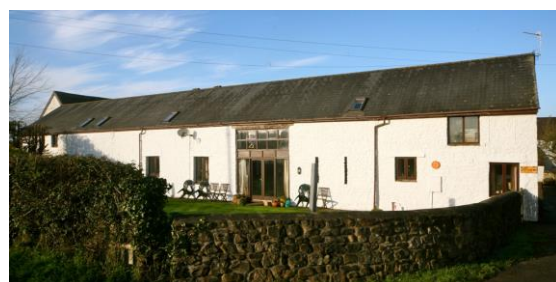
Fig.18 Swallows Nest barn, a long threshing barn at Clytha Farm
