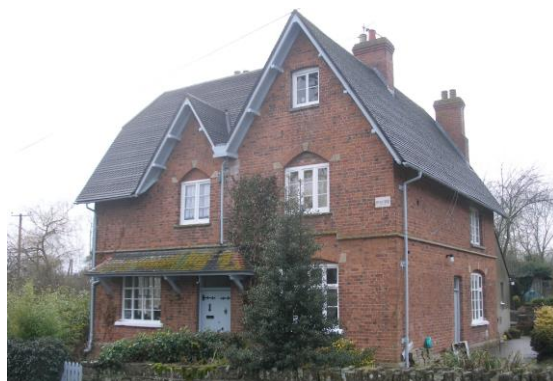
Fig.62 Bryn Teg. A particularly fine pair of High Victorian houses in Llanarth village. The reinterpretation of farmhouse architecture suggests a fusion between the revivals of both Gothic and vernacular styles.
