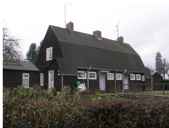
Fig.66 Numbers 1 and 2 Plas yr Haul, Great Oak dating from 1939. A pair of estate cottages contrasting with its neighbours has dark stained timber cladding and a tall distinctive gambrel roof.
