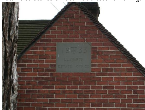
Fig.67 Red brick is a characteristic of early to mid 20 th century estate buildings
