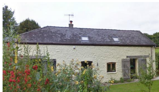
Fig.77 Coach House, a converted stone barn opposite Beech House
